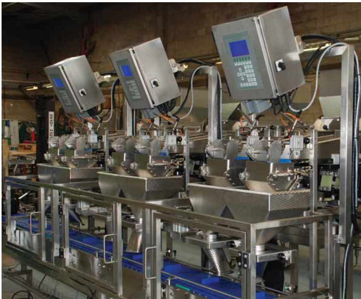
Pulling out all the stops: Cotswold Mechanical was up against a tight deadline to complete the project for Hider Food
